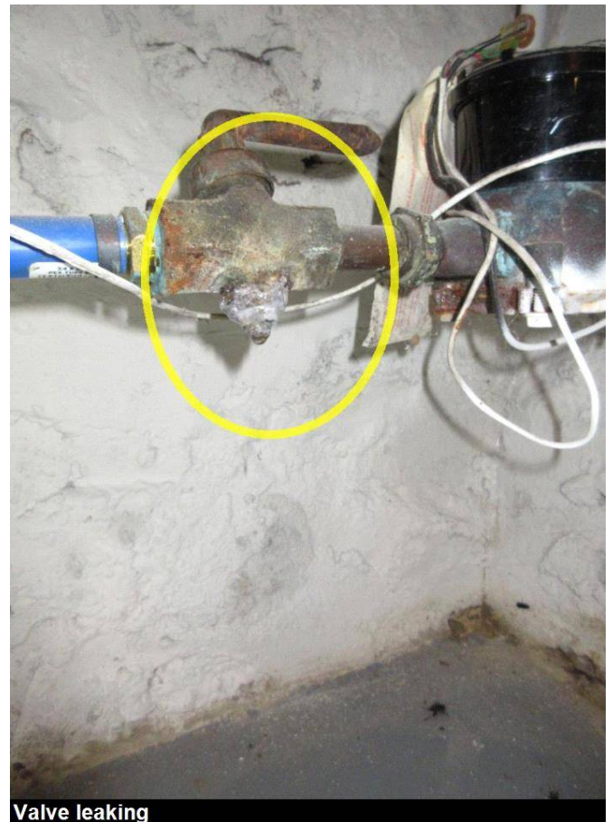
Valve leaking
